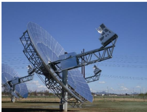
Figure 1.20 Maricopa Dish-Stirling plant 1.5 MW, Arizona, USA (left); parabolic dish system plant schematics (right)
